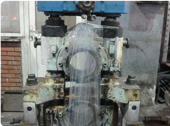
Rebars rolling mill stands
