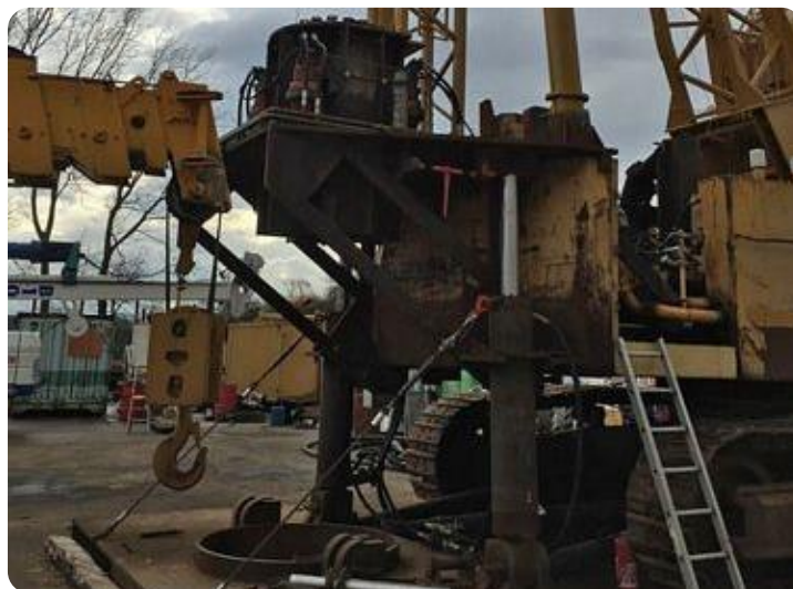
Head of a drilling rig
