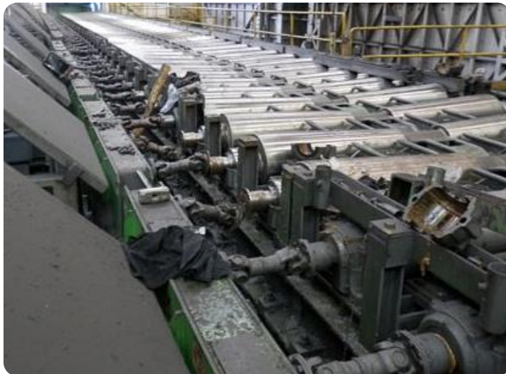
Run out table on hot rolling mill
