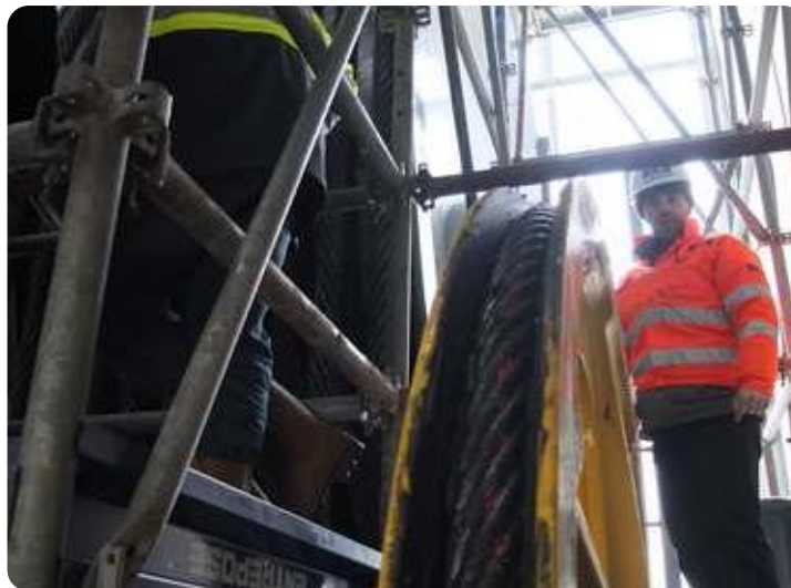
Pulley of a bridge lifting mechanism
