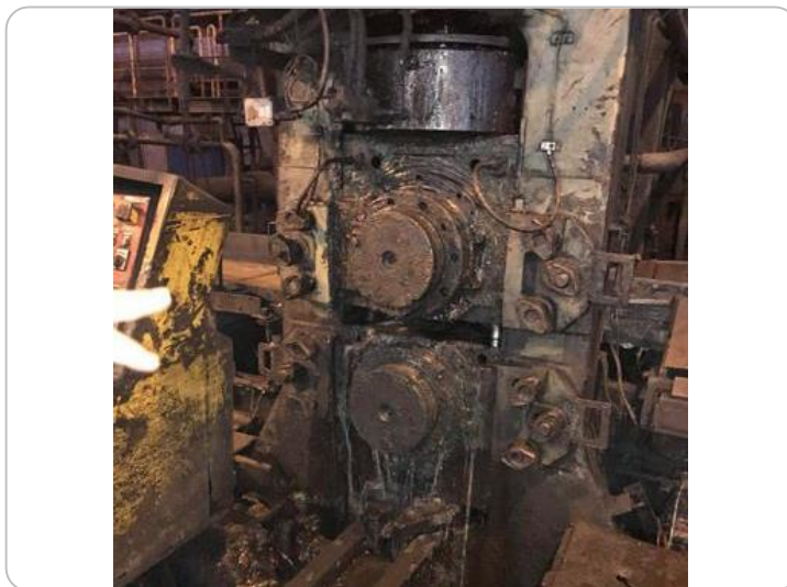
Hot rolling mill line
